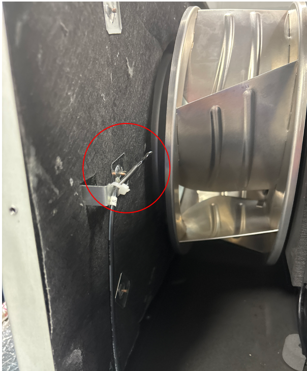
Figure 409 (Indoor Coil Temp. Sensor, T2) To access the evaporator coil sensor remove the top panel and right side upper panel.
