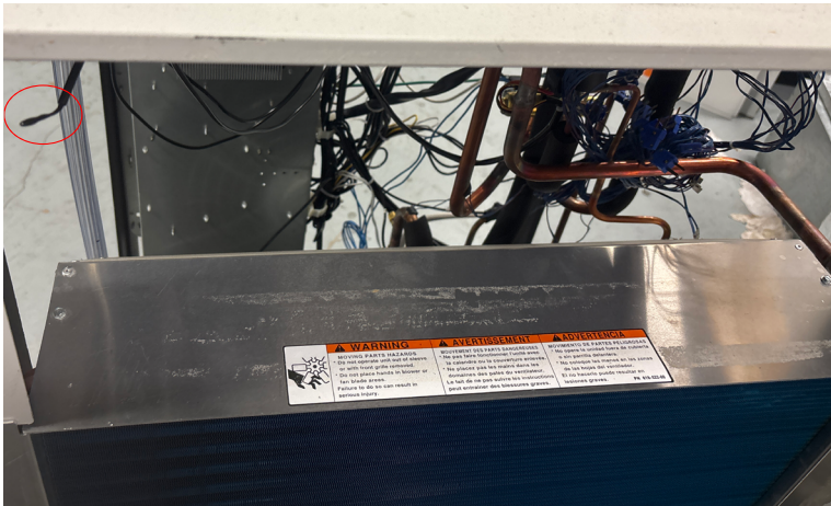
Figure 405 (Outdoor Ambient Air Sensor, T7) is located in the outdoor section, mounted on the bottom of the indoor blower housing.
