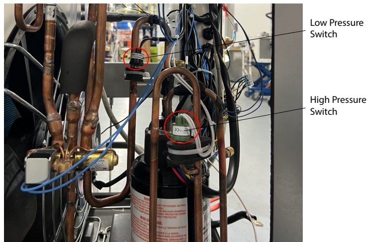
Figure 425.1 (Pressure Switches)
