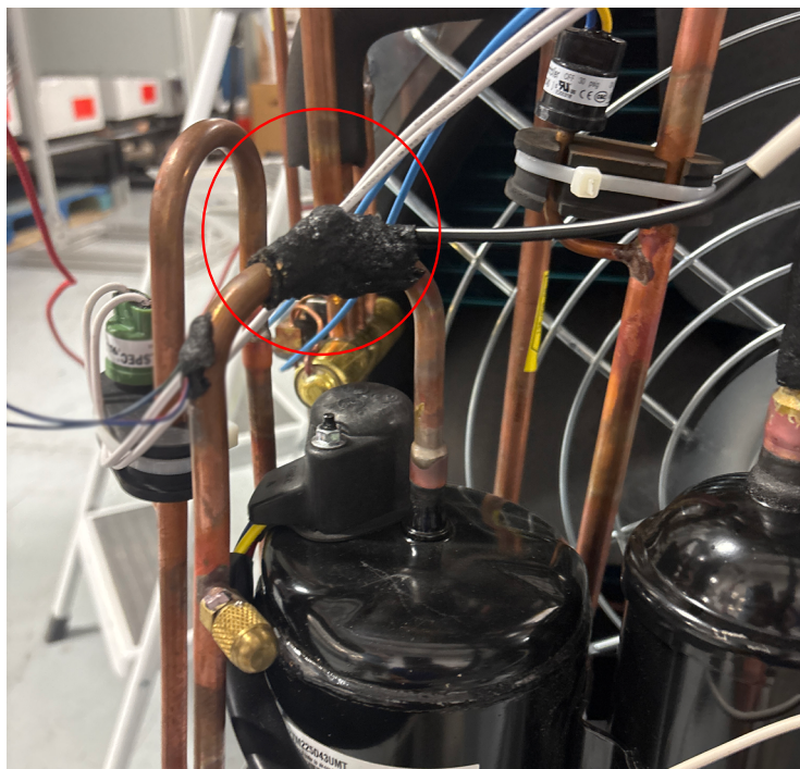
Figure 407 (Compressor Discharge Temp. Sensor, T4), located on the compressor discharge line.
