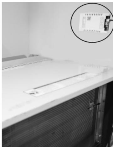
Mount the Receiver as high as possible. It MUST be higher than the VRP unit (top)
