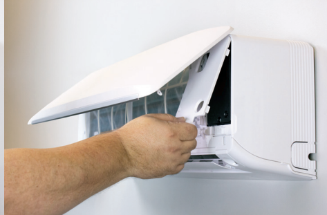
Remove electrical access panels (2)
