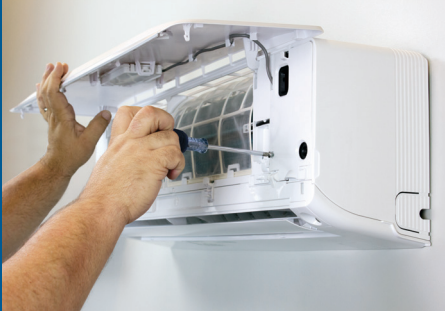
Back out electrical panel screws
