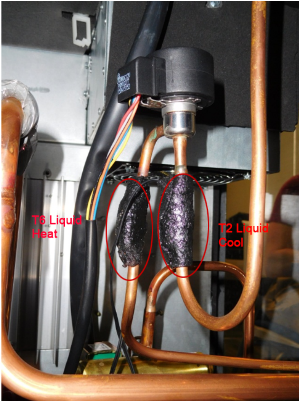
Figure 628 (Thermistor Locations)
