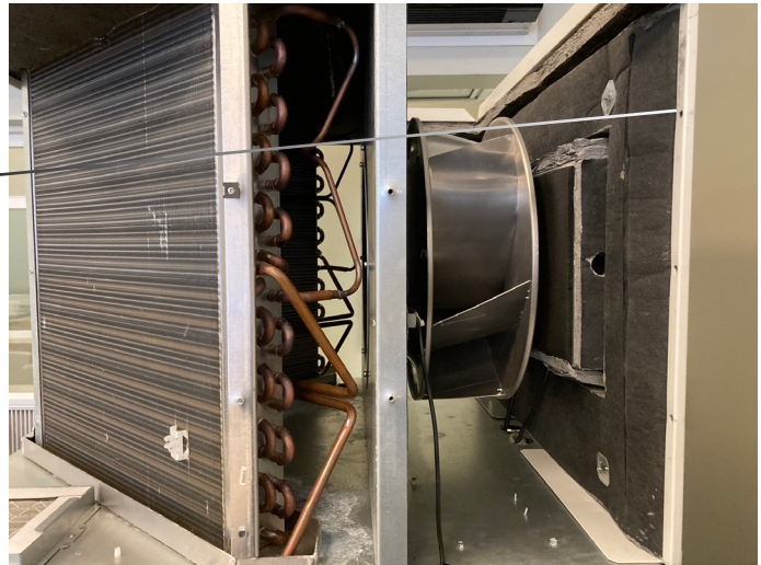
Figure 507 (Support blower panel)
