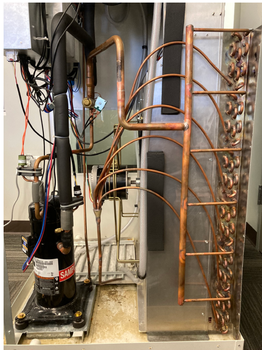
Figure 504 (36k Condenser replacement)
