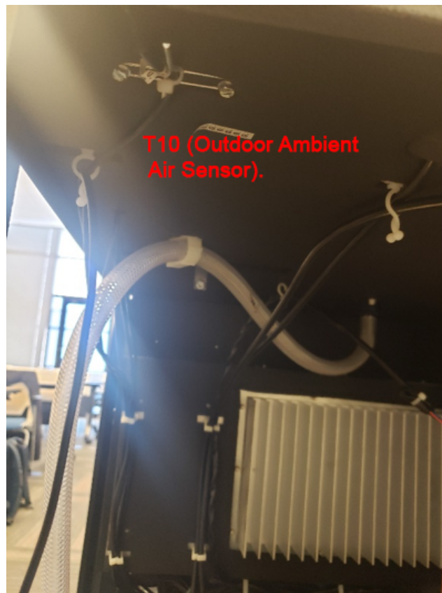
Figure 629 (Thermistor Locations)
